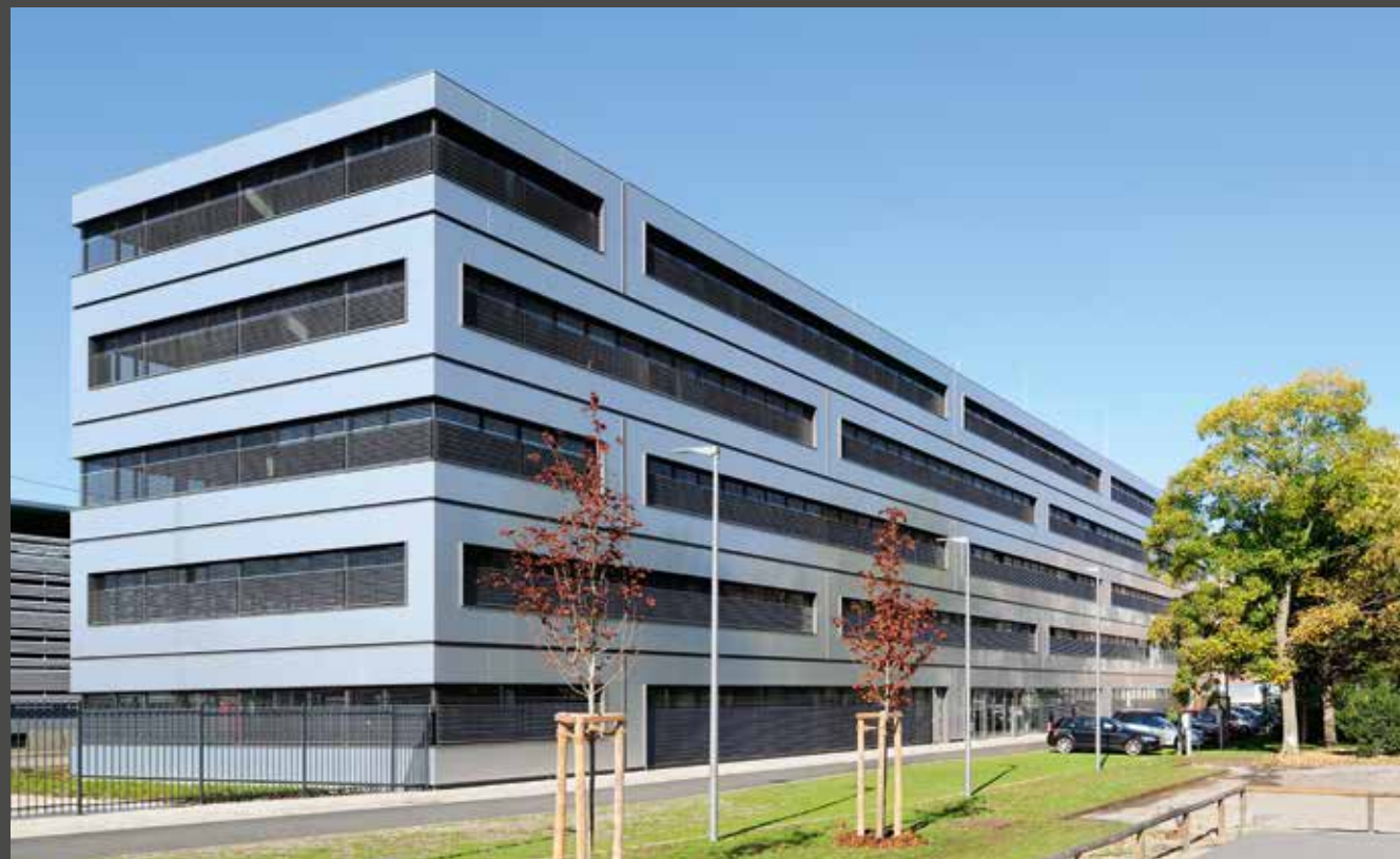
Technopark Siemens AG, Nuremberg, Germany | Architect: Brückner & Brückner Architekten | Material: ALUCOBOND® naturAL Brushed | © Ralf Dieter Bischof
